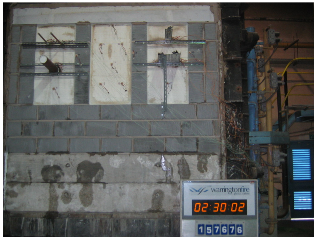
The unexposed face of the assembly after 150 minutes of testing
