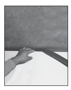
Foam is simple to install for head of wall applications. Compress the Blaze Foam into the joint between the top of the wall and bottom of the deck so that the intumescent strip is facing the wall surface. Blaze Foam can be recessed into the joint or installed flush with the outside surface of the wall. Joints are butted together. No mechanical fastening of Blaze Foam is required.
